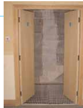
Internal door smoke and heat exhaust ventilator (AOD)
