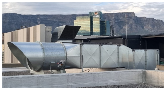
Top of Shaft Roof Mounted Powered Extract Fan
