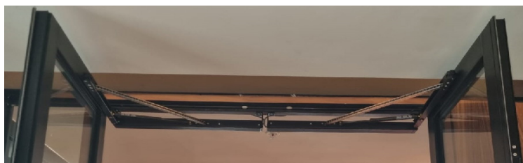
SECO Ni Folding Arm Actuators provided precise operation of doors utilised for smoke ventilation within the office areas of the building
