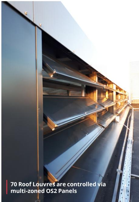
70 Roof Louvres are controlled via multi-zoned OS2 Panels
